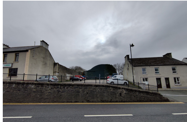
Existing Cope Yard, Creeslough © Arup
