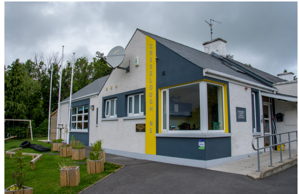
Creeslough National School © Arup
